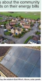
Top, the estate in East Winch. Above, solar panels.
